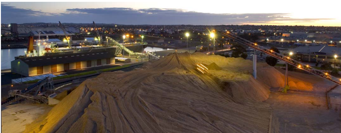
Midway facility, Port of Geelong Source: Les Branch, Midway Ltd
