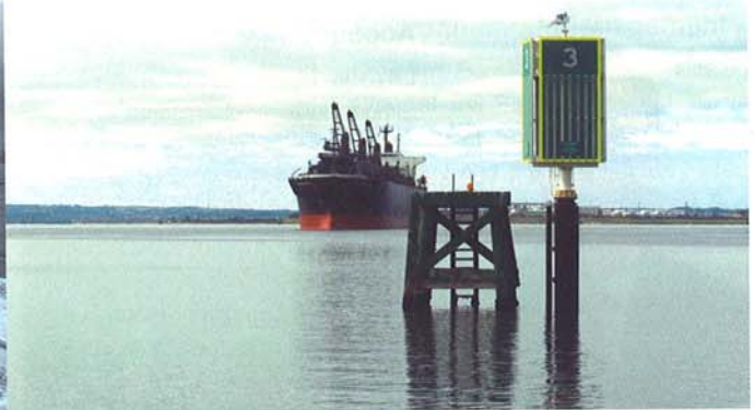
New navigation beacons have been installed along Corio Bay's shipping lanes.
